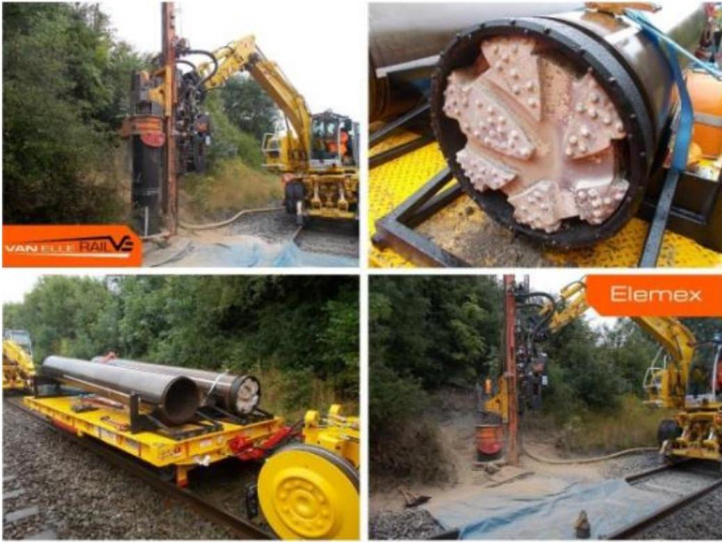
**Figure 5-3: Drilled permanent steel pile OHLE foundation solution option (source Van Elle)**
