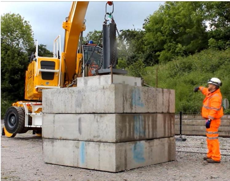
**Figure 5-4: Precast ground bearing pad foundation and micro-pile solution (source Van Elle OHLE SmartBase)**
