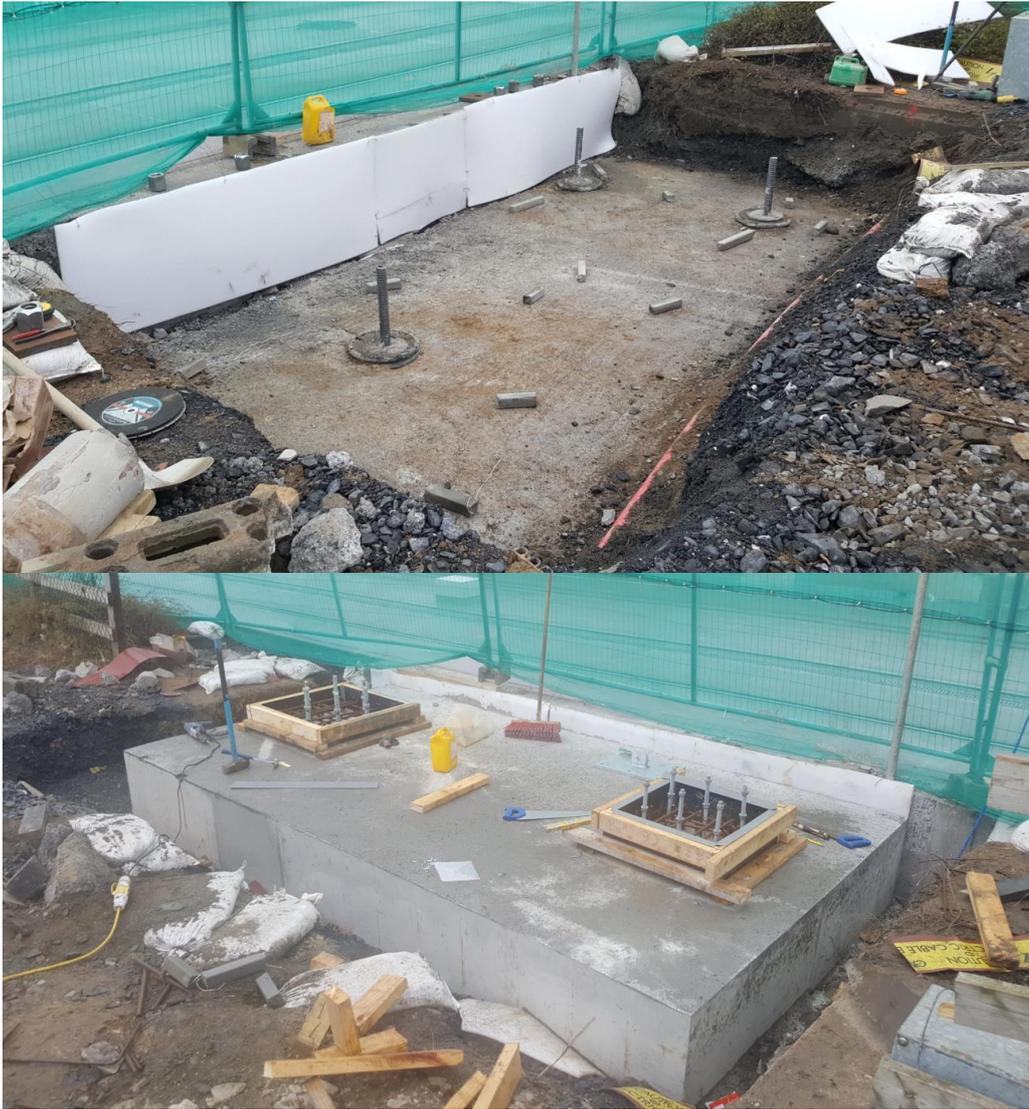
**Figure 5-5: Mini-pile foundation solution; *top*; three-pile group following piling works and placement of concrete blinding, and *bottom*; foundation following construction of the reinforced concrete pile cap. (source Arup)**
