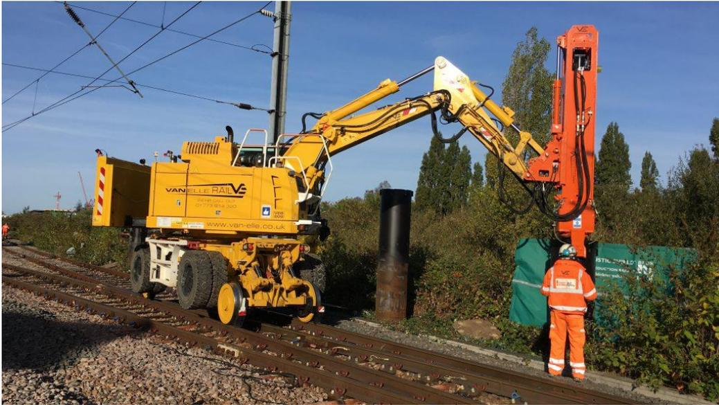
**Figure 5-6: Driven (circular hollow section) steel pile installation (source Van Elle)**
