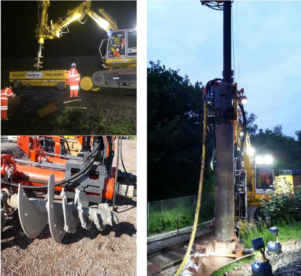
**Figure 5-2: Example of a rail mounted rotary bored piling system; *left*: auger type drilling equipment, *right*: percussive down the hole hammer drilling equipment (source Arup)**
