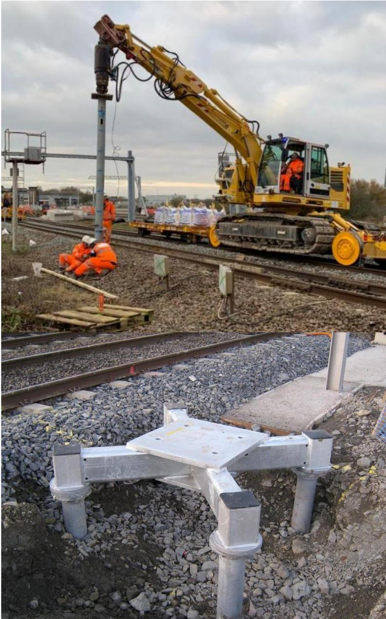
**Figure 5-7: Screw pile foundations for OHLE; *top*; screw pile installation (source Van Elle), and *bottom*; four pile group screw pile foundation (source IÉ)**
